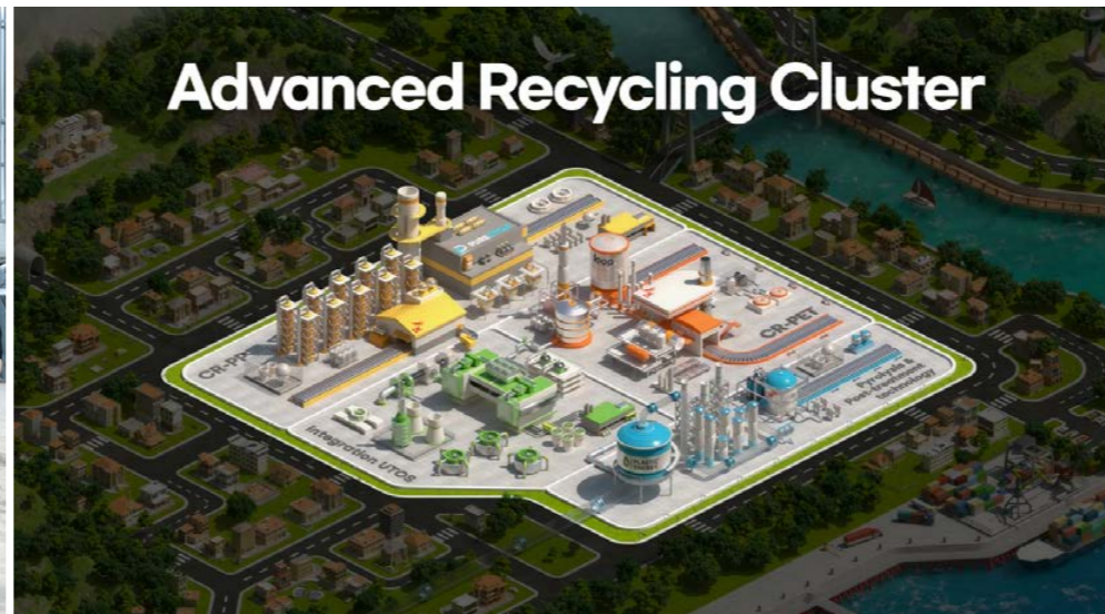
Advanced Recycling Cluster under Construction by SK Geo Centric
