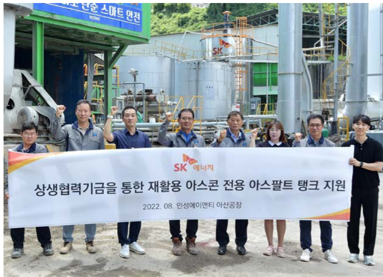
SK Energy and Inseung A&T complete the construction of an asphalt tank exclusive to recycled asphalt concrete
