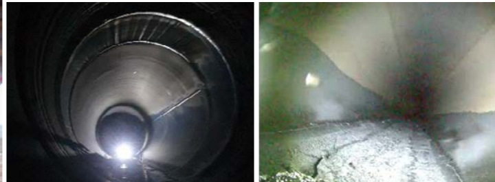
Inspection of the inside of pipelines at the Ulsan CLX of SK Innovation (robotic snake)
